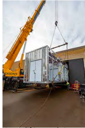
Crane lifting pods into the existing warehouse dock door.
