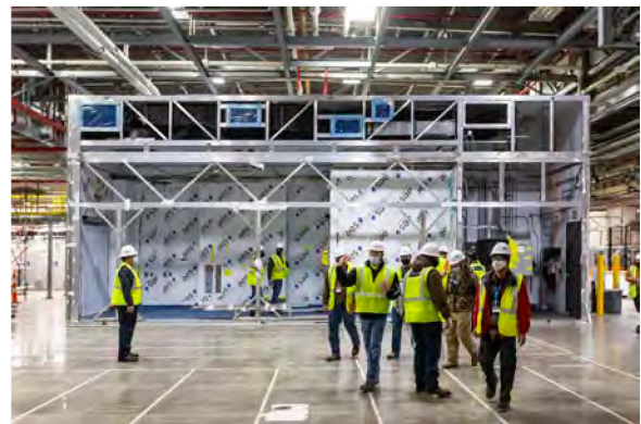
Image showing aluminum trusses of single section pod allowing for open clean room span.
